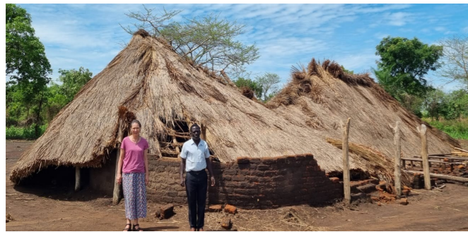
The original St. Luke's Church damaged by a storm.
